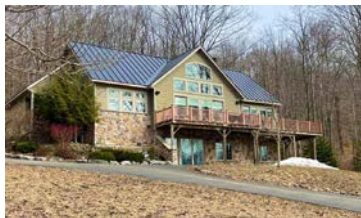
6876 Leslie Road. $709,000 Gorgeous home! 2 mins. from the slopes. Amazing views! 4 bdrm 3 bath 2,731 sq ft
