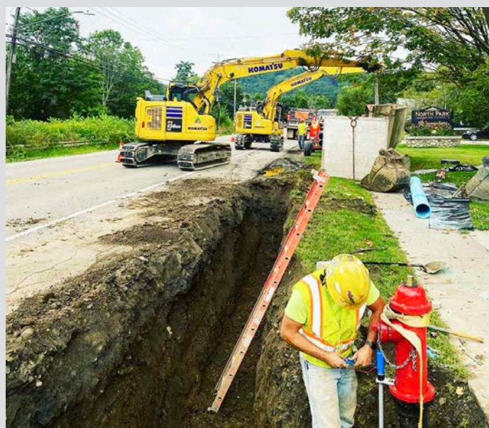
jd_northrupconstruction: Water Main replacement. #ellicottvilleny
